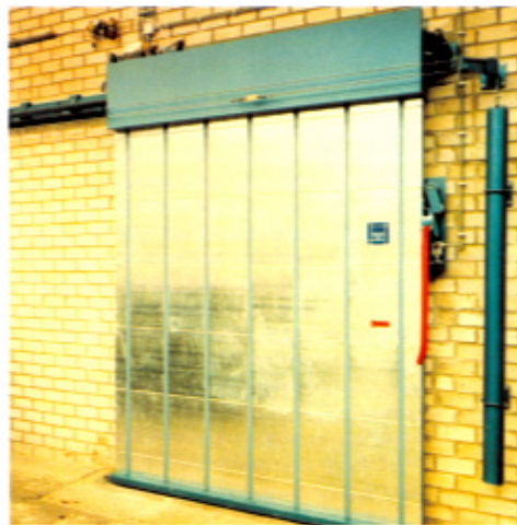
M2-BR 360 (above) 6 hour sliding fire door with pneumatic opening device
