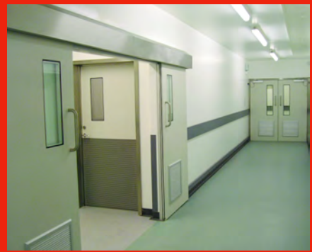
GRP doors in typical Hospital
