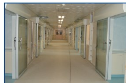
With 2 x 6mm thick hardened glass, flush fixed with anodised aluminium door blades, these MF5 hermetically sealing glass doors maximise natural light
